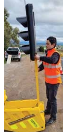
Extend the mast Pull knob out and raise.
